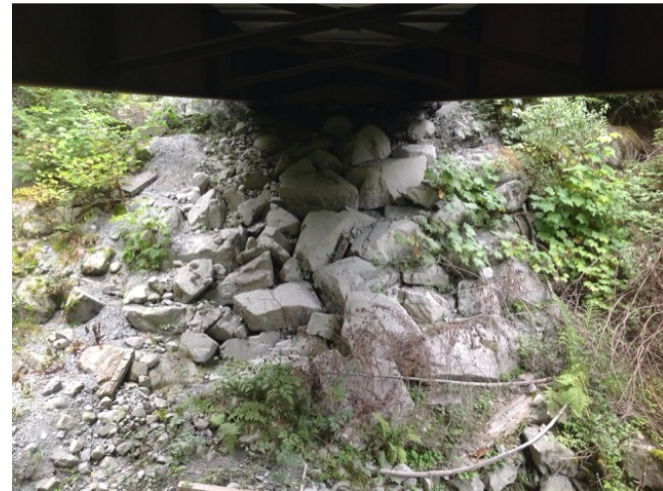
Left Bank Abutment when facing downstream
