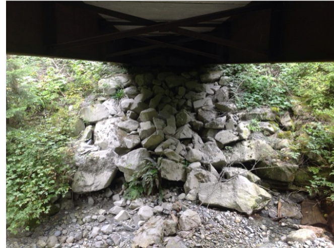
Right Bank Abutment when facing downstream
